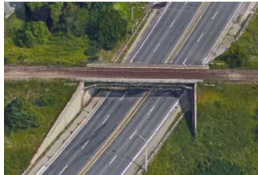
Exhibit 8.1: CN Rail Crossing of Highway 2 in Pickering
