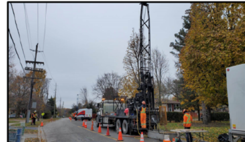
Figure 1: YNSE Geotechnical Investigations
