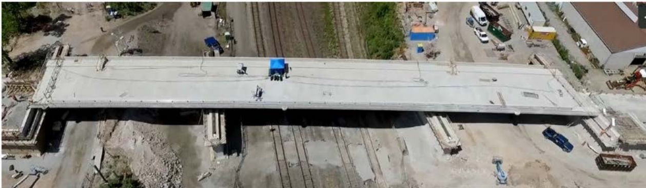
Lifting & Moving of Kodak Building, Crosstown Mt Dennis Station
