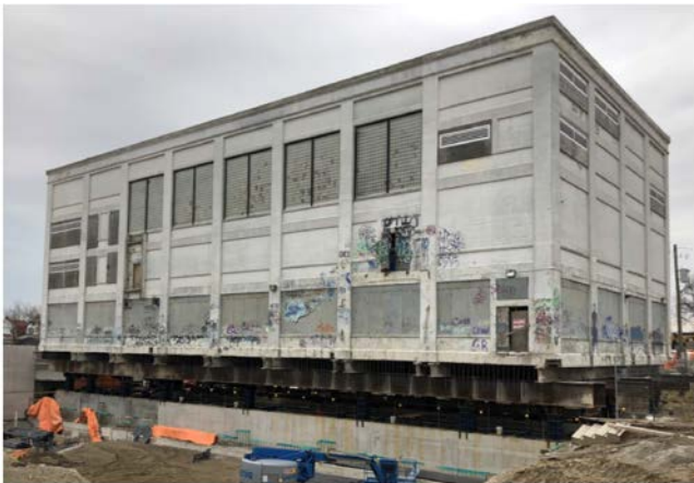
Eglinton Station - Subway Support Risk Management
