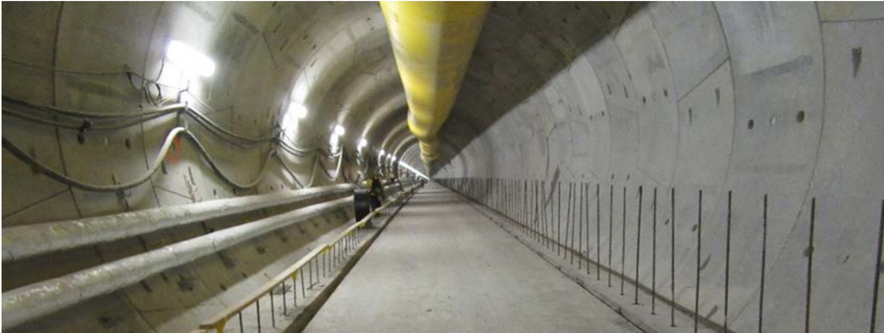
Eglinton Crosstown Tunnel, Segment 6, Concrete poured, and ready for track installation, July 27, 2017.
