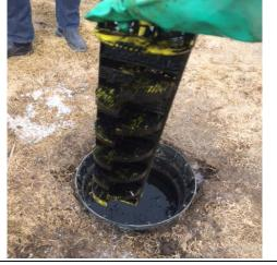
5 Elevated effluent level in septic tank
