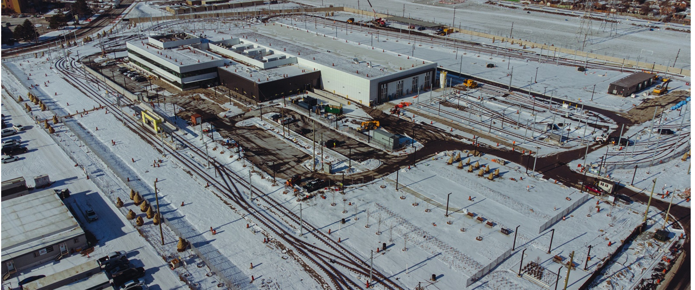
Photo: Aerial view of Maintenance and Storage Facility.
