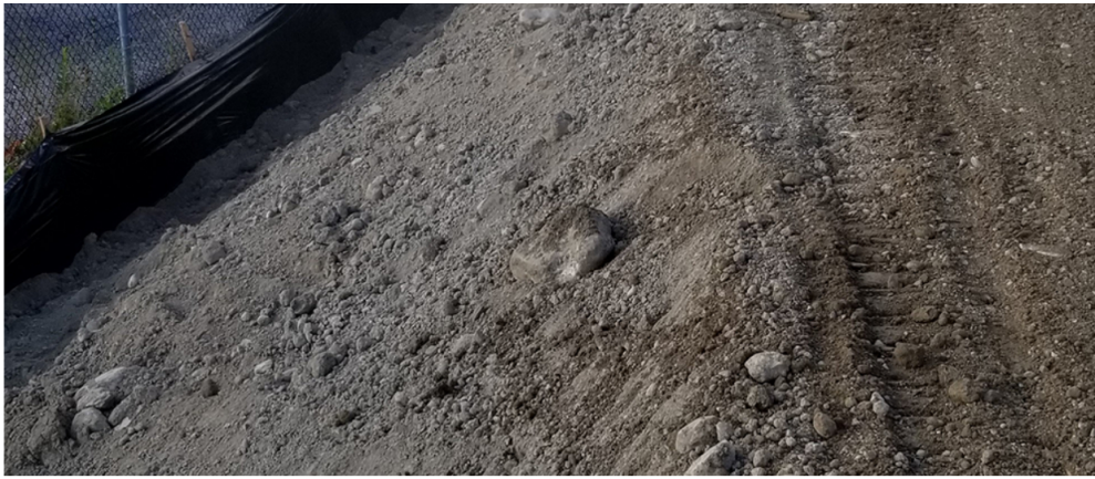
Example of silt fencing used for erosion and sediment control
