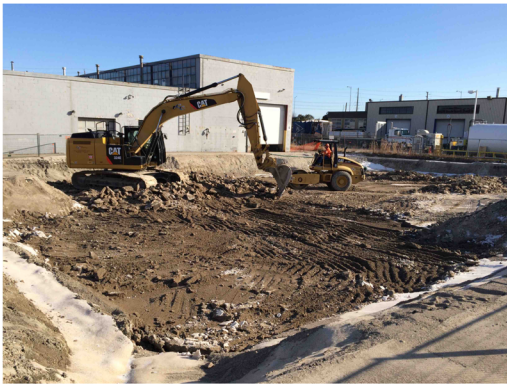
Asphalt removal on a construction site. Source: AECOM, 2016.
