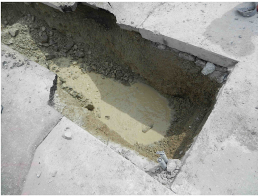
Asphalt removal on a construction site, revealing groundwater. Source: AECOM, 2016
