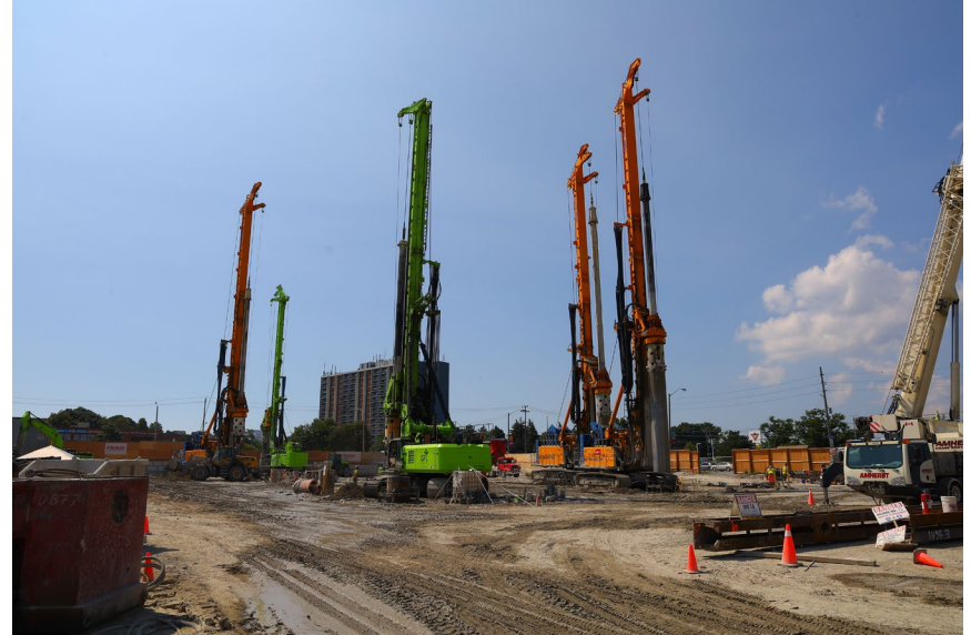
Drill rigs at the launch shaft site at McCowan and Sheppard. Piling at this site is complete.
