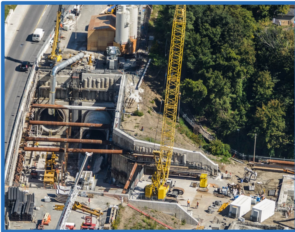
(2016)Launch shaft for Crosstown LRT TBMs
