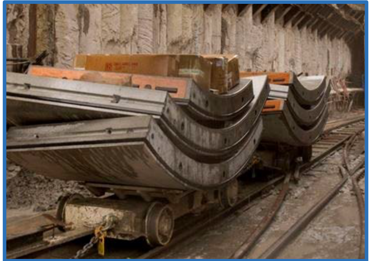
Crosstown LRT precast tunnel liners
