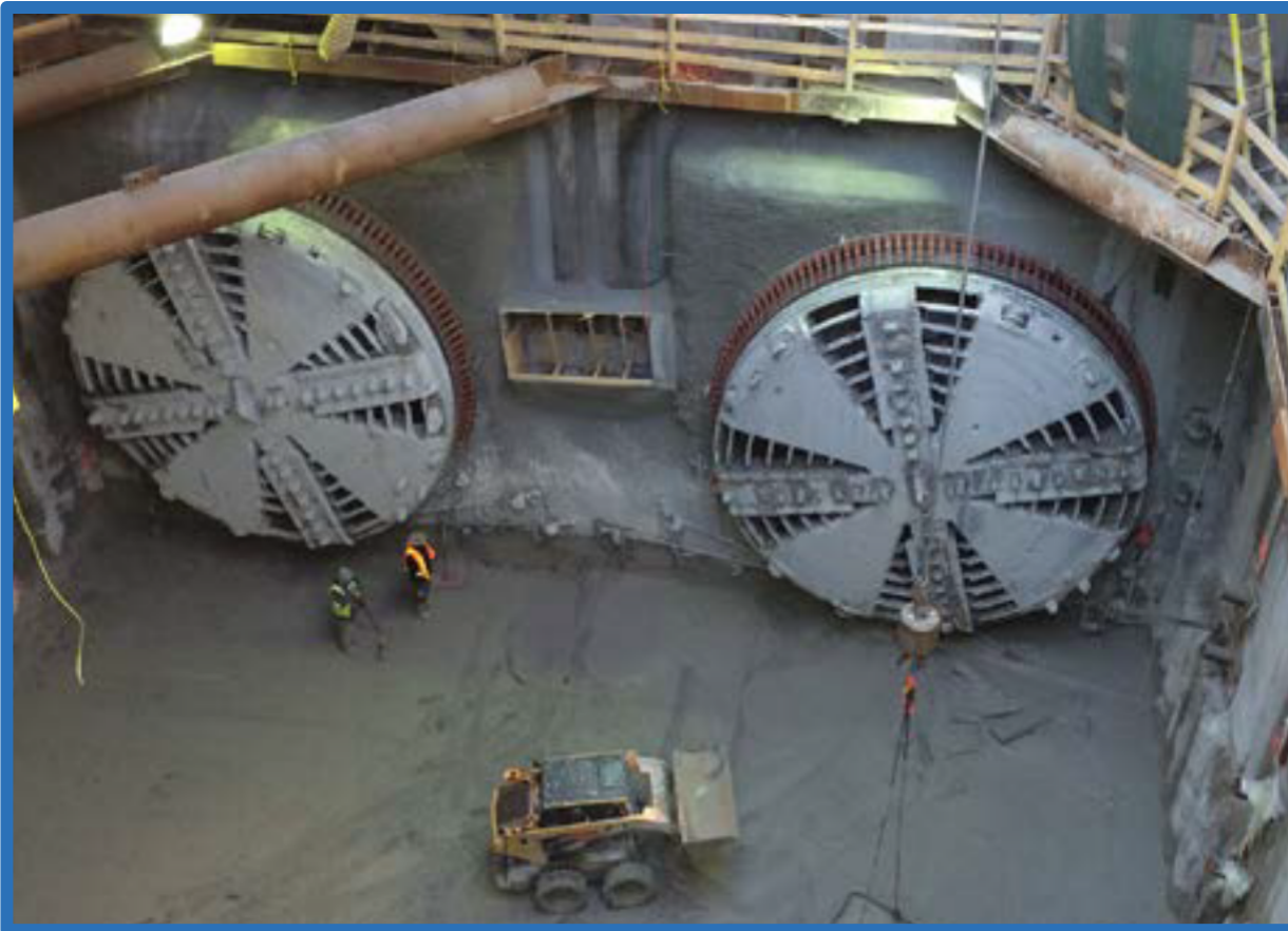
Crosstown LRT tunnel boring machines
