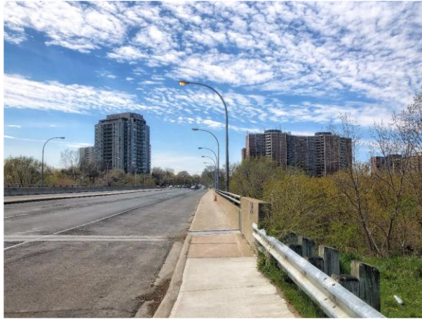
Looking west along the Eglinton Ave. bridge
