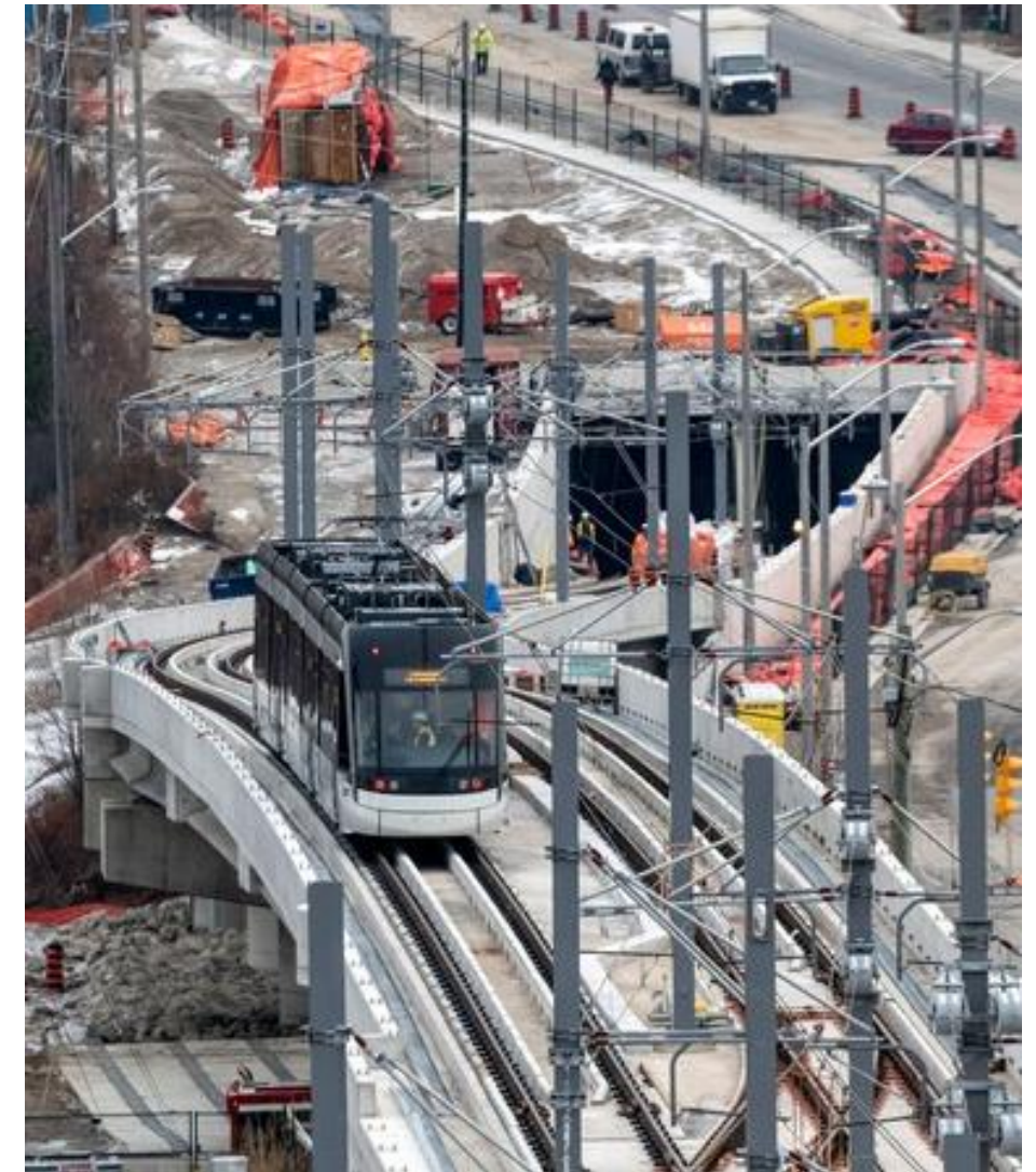
Crosstown LRT portal at Black Creek Dr.
