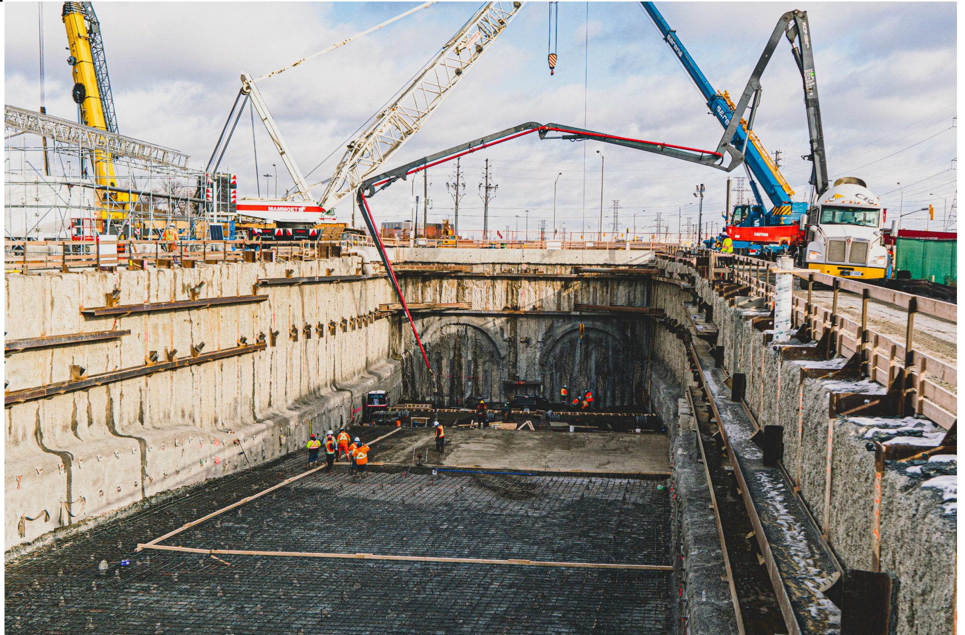
TBM launch shaft excavation progress at Renforth Avenue (Dec. 2021)
