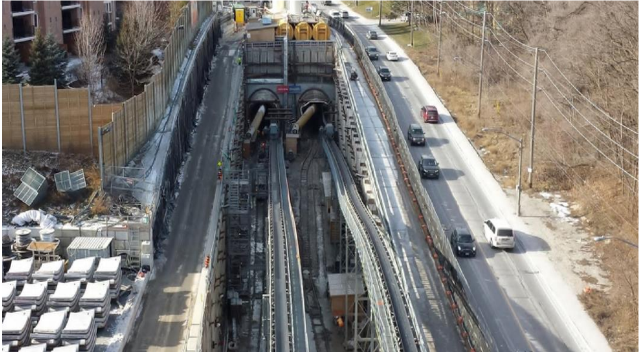
Figure 2-3 Typical Portal Structure, Under Construction
