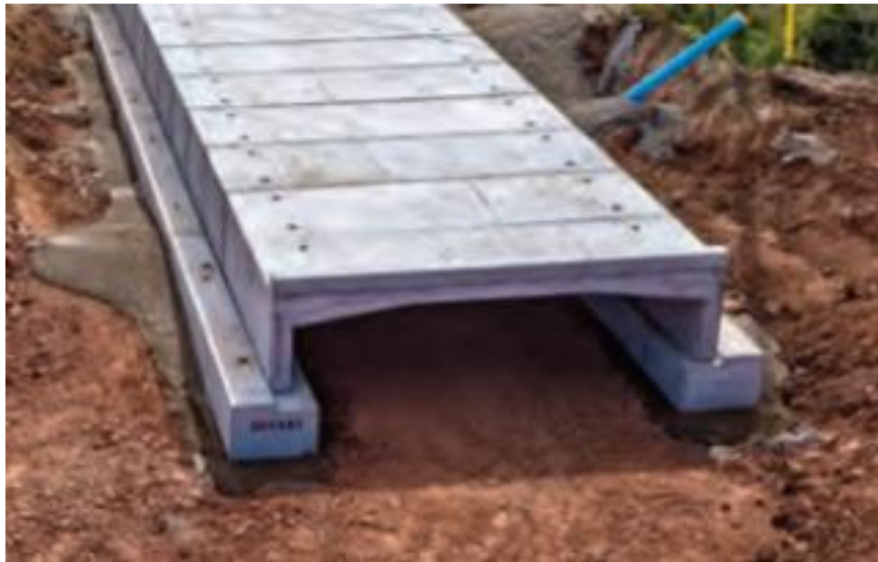
Figure 5-7 Typical Modular DECAST Culvert
