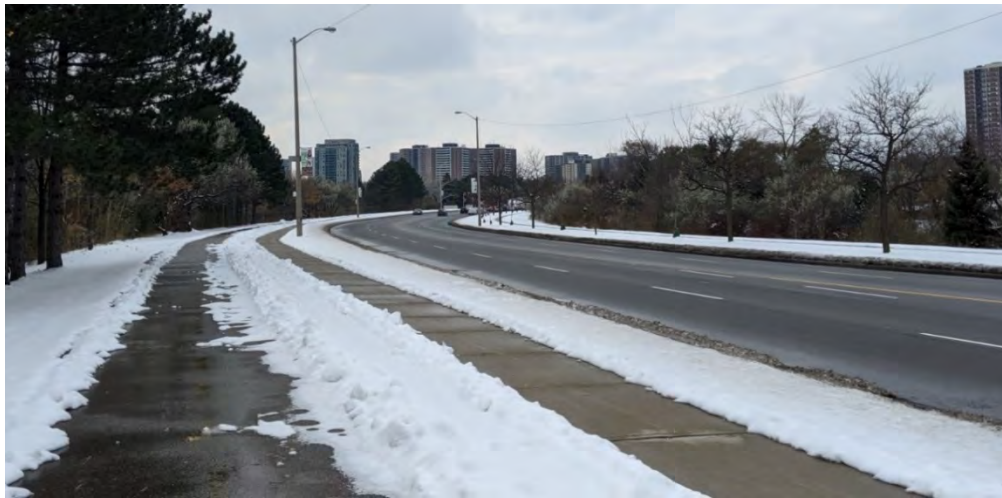
Figure 3-3: Eglinton Avenue West, Looking West, West of Jane Street 19
