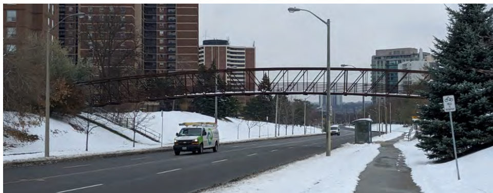
Figure 3-1: Existing Pedestrian Bridge West of Scarlett Road 17
