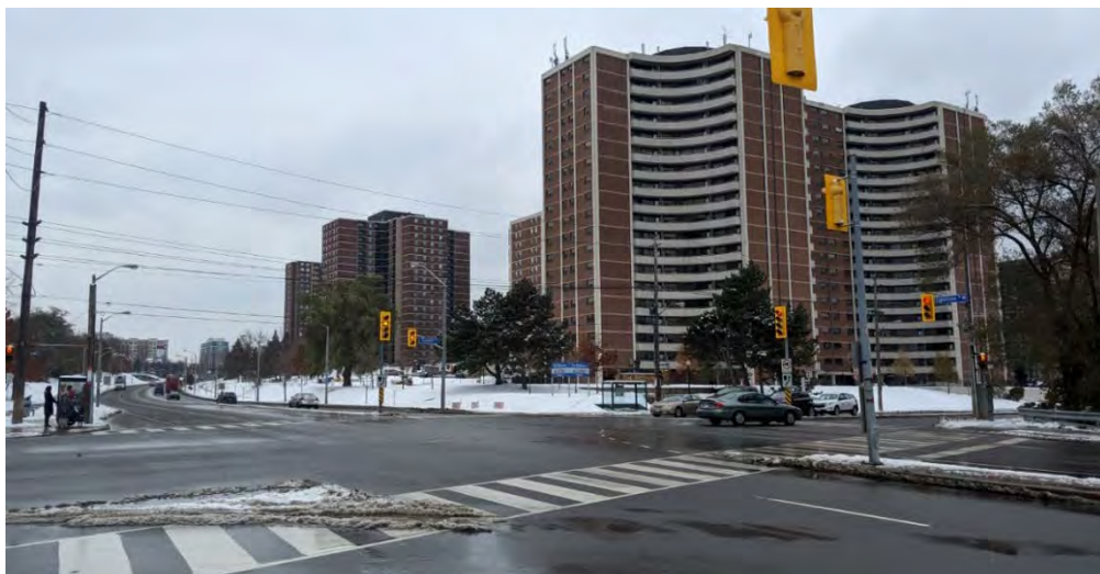
Figure 3-4: Eglinton Avenue West and Scarlett Road Intersection, Looking West 20
