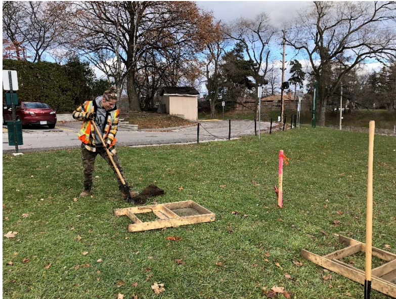
Photograph 7-31: Looking Northeast at Crew Test Pitting at 5 m Intervals
