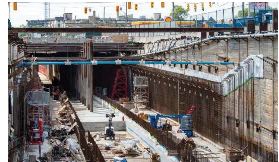
This view is looking under the Kennedy and Eglinton intersection, with formwork in place for more concrete pours.
