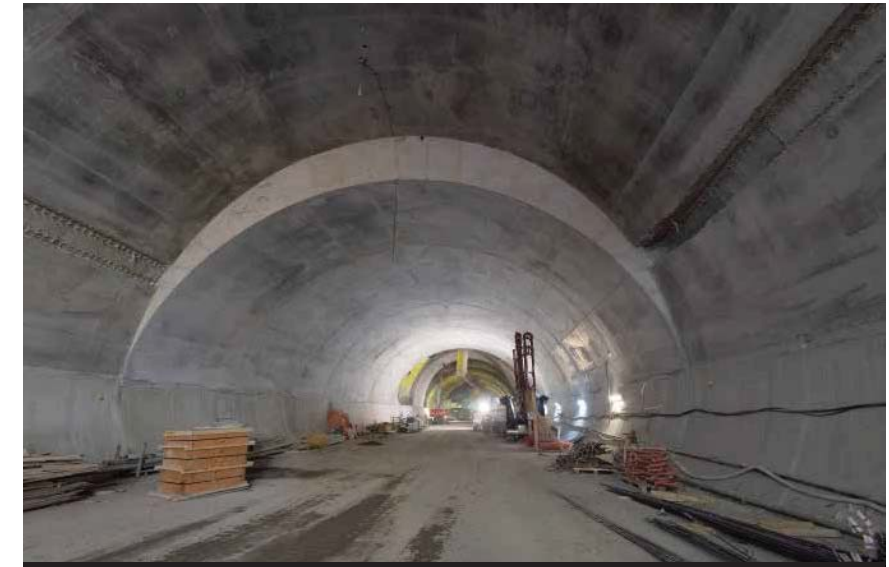
This view shows the mining at Laird Station, with completed sections of floors and roof archway.
