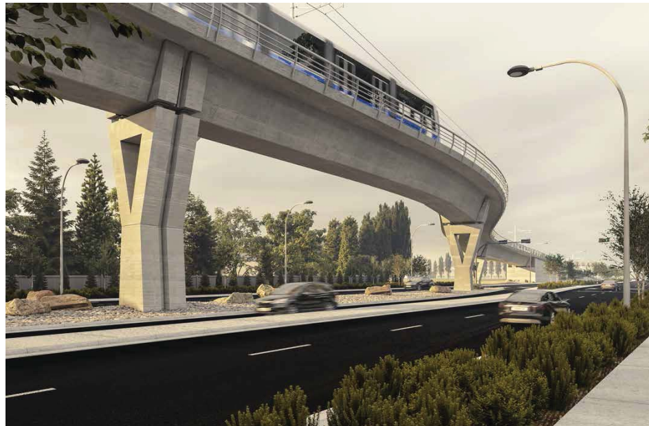
Valley Line LRT, City of Edmonton
