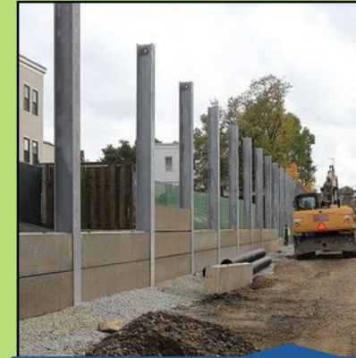
Noise/Retaining Wall Installation (Aug 2022)
