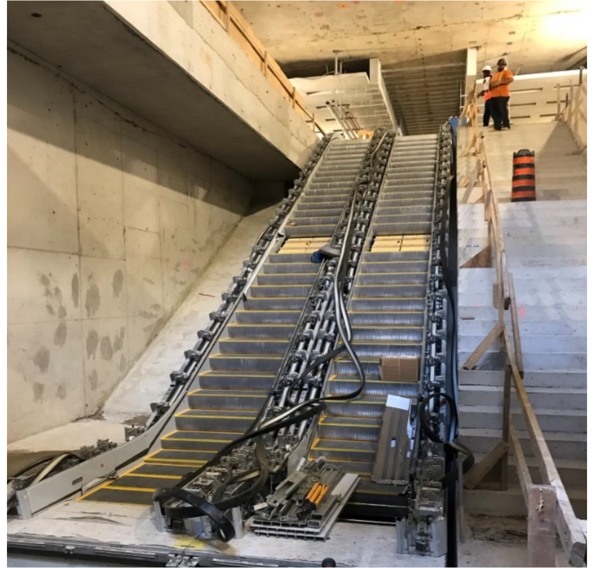
Photo: Escalator installation in Finch West Station. 2022.09.21
