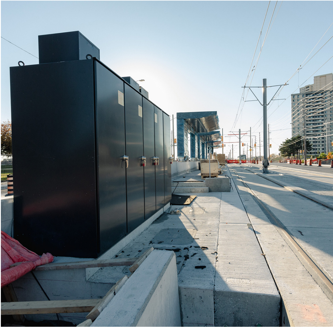
Photo: Electrical cabinets installed at Driftwood platform stop. 2022.10.28
