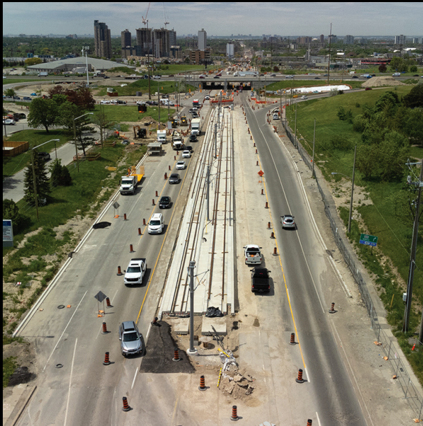
Photo: Westward view of the track slab, from Norfinch Avenue to Highway 400.
