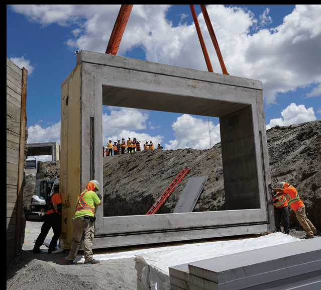
Photo: Placing the first precast piece of the tunnel.
