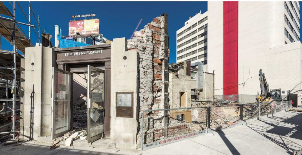
Mount Pleasant during construction (December 2021)
