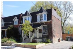
15 and 17 Tiverton Avenue. Source: AECOM, 2020.
