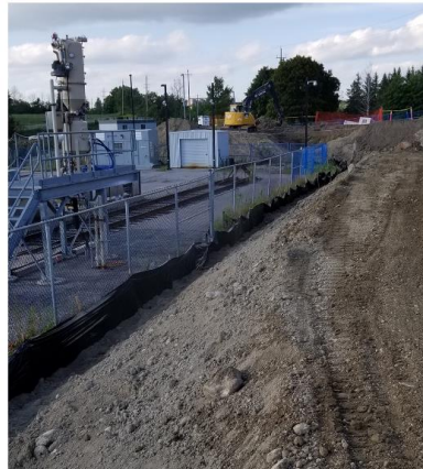
Example of silt fencing used for erosion and sediment control. Source: Metrolinx, 2020.
