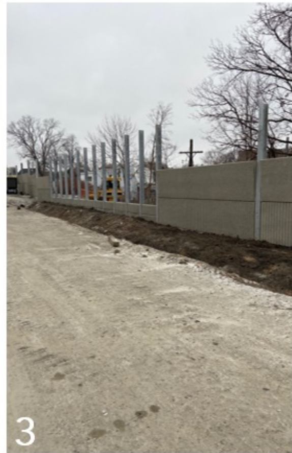
3 & 4. Noise Barrier Wall Construction
