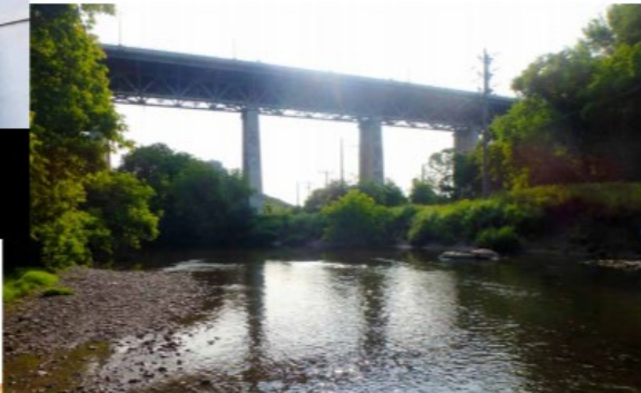
Millwood Road Overpass Bridge crossing the Don River
