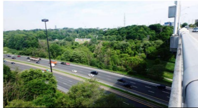
Crossing of the Lower Don River Valley at Millwood Road Overpass Bridge
