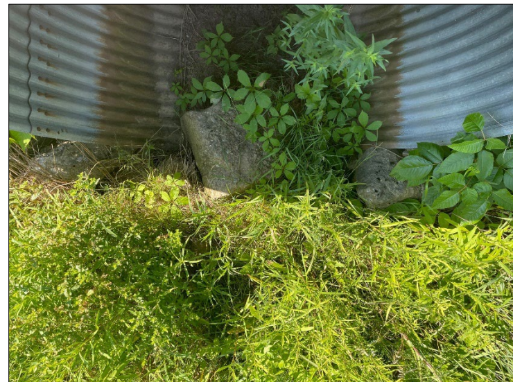
Upstream end of east culvert
