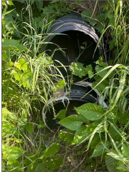
Downstream end of culvert
