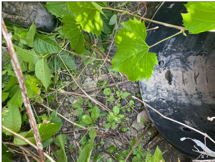
Upstream end of culvert
