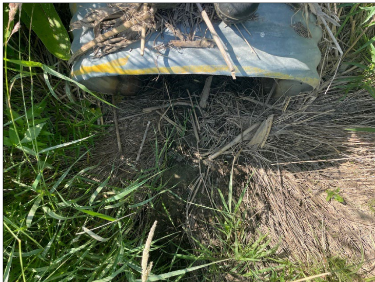
Upstream end of culvert
