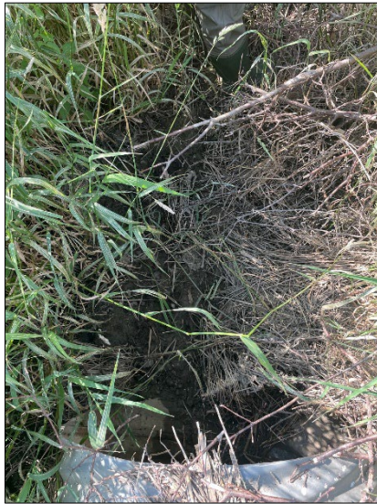
Downstream end of culvert
