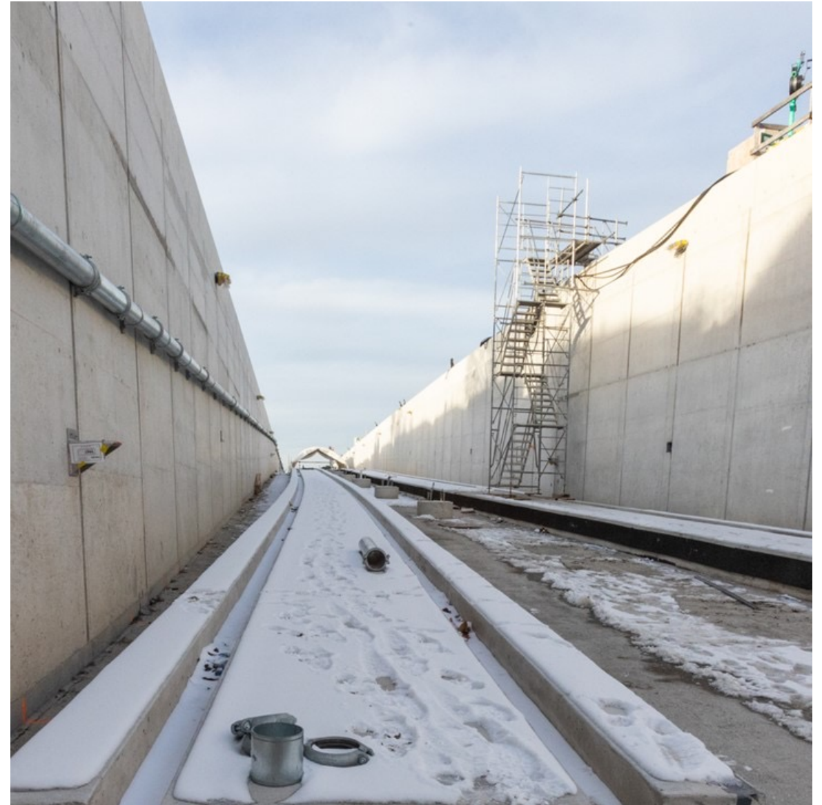
Photo: Humber College Station Portal Track slab . 2022.12.14
