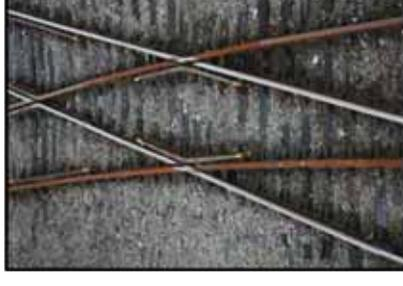
Standard crossover or frog showing gaps between the rails that generate additional noise and vibration
