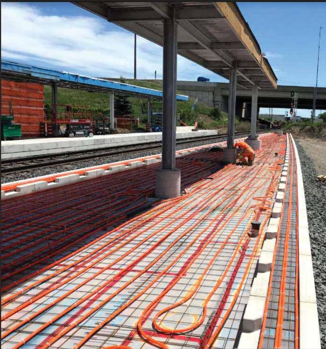
At Unionville GO, crews are installing the snow melting system to maintain safe walking conditions for customers at the platform. In the east platform, soffit panel installation is underway at the canopy, while formwork for shelter cubs continue to take shape on the west platform.
