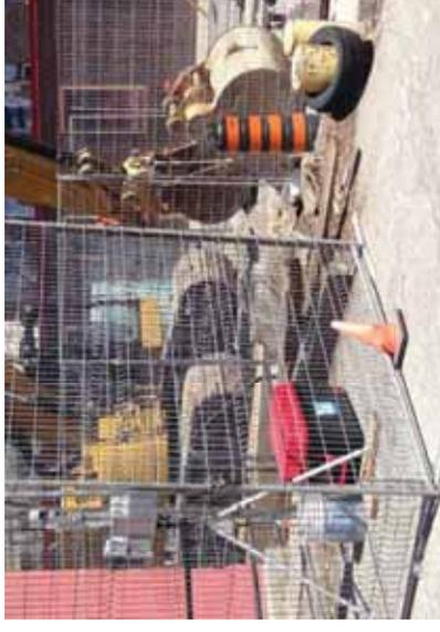
Example of construction dust monitor in a fenced enclosure (left side of photo)
