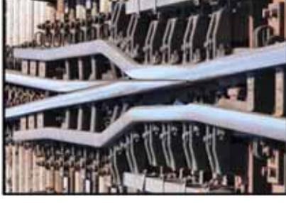
Moveable point frogs eliminate the gap between rails at crossovers, reducing the noise and vibration from trains passing over those crossovers
