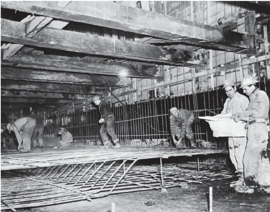
1950 – Workers install concrete rods to reinforce concrete that will be poured to support the underground tunnels as they work to build the Yonge line – Canada’s first-ever subway. (Image courtesy of the Toronto Transit Commission)
