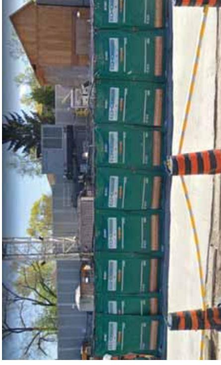
Example of moveable construction noise-absorbing barrier.
