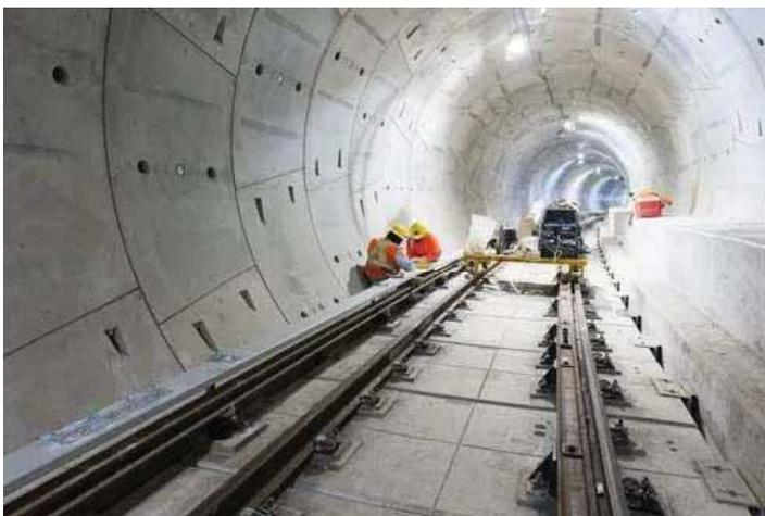
The tunnels along the western leg of Line 1 are built with floating slab subway track, a modern design innovation that reduces noises and vibration as trains pass over them. (Image courtesy of
