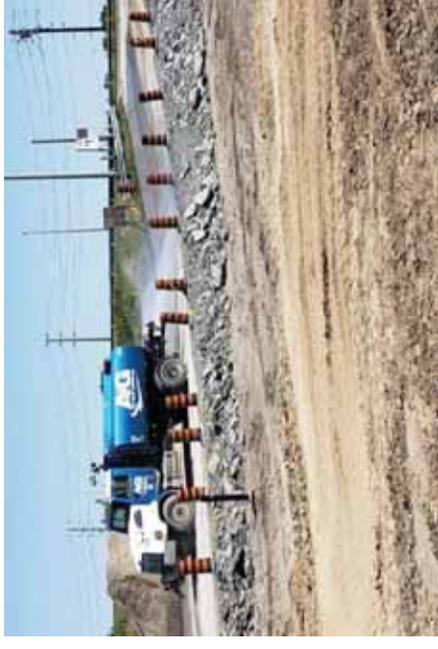
Example of watering truck used for dust suppression
