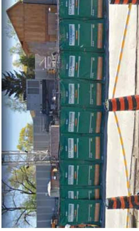
Example of moveable construction noise-absorbing barrier.
