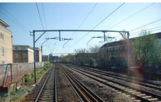
Figure 3-4: Typical Overhead Contact System (OCS) Infrastructure in an Urban Setting
