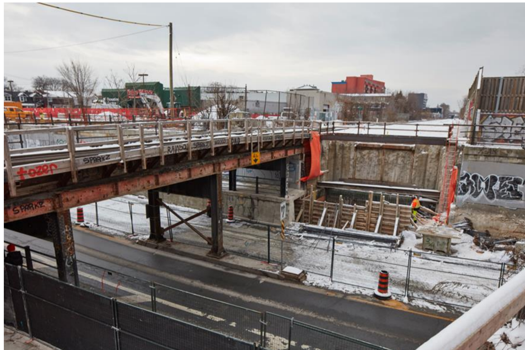
South bridge abutment construction (looking south).
