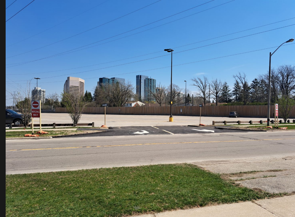
Excavation work around utility and TTC underground structures (Top) and Completed Talbot Road Temporary Exit (Bottom)
