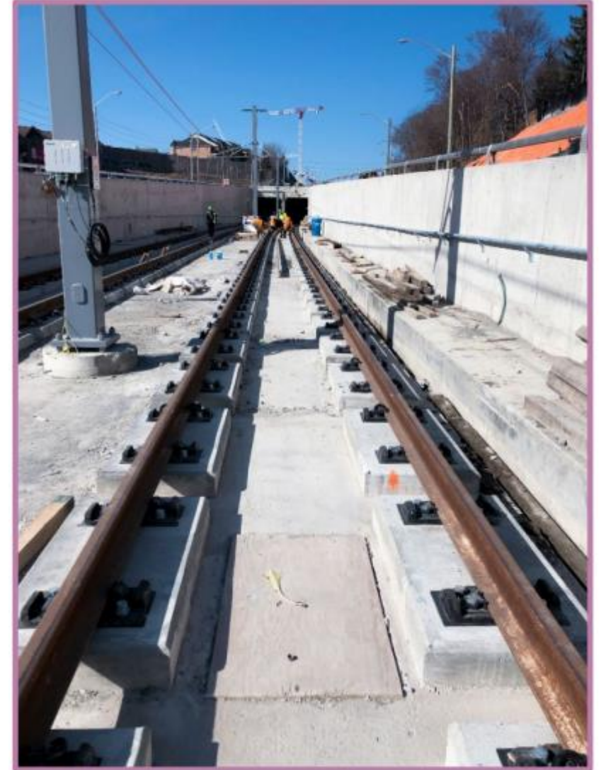
Crosstown LRT east portal (2021)
