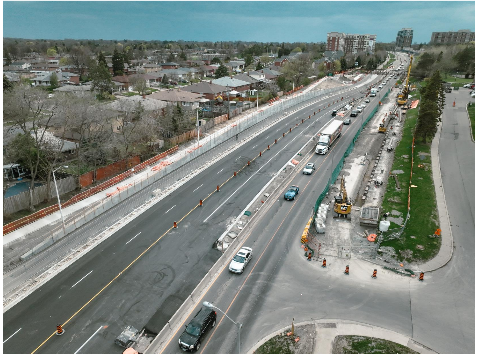
The extraction shaft site in April 2023 - Road realignment work
