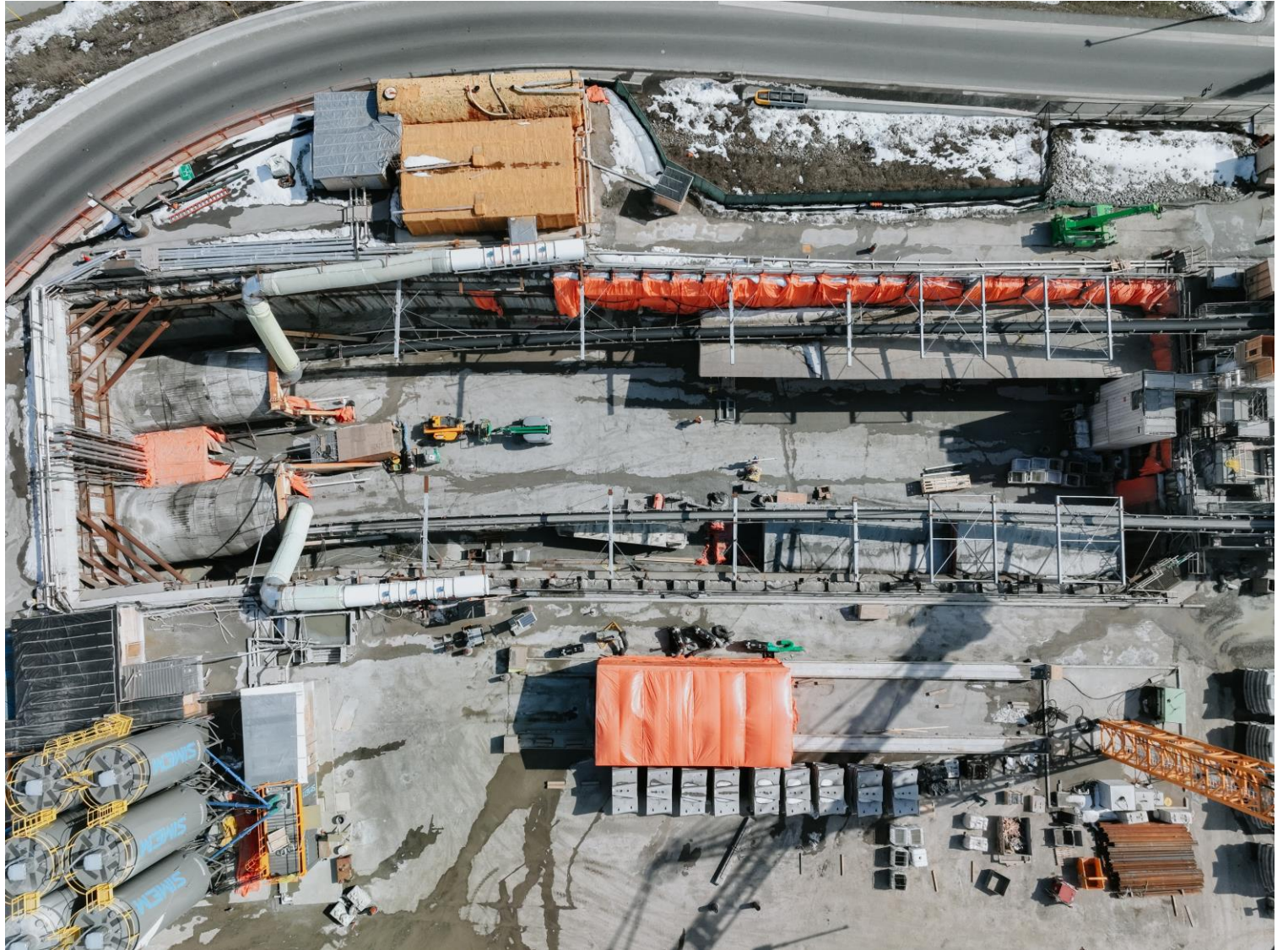
The launch shaft in March 2023
