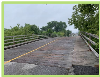
Albert Street Bridge
