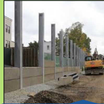
Noise/Retaining Wall Installation (Jan 2023)
