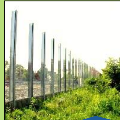
WTRP Realignment (March 2024) Ph3 Pedestrian Diversion
