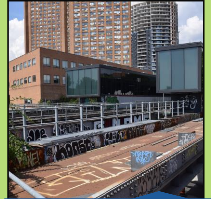
Bloor St Bridge Shift (Spring 2023)
