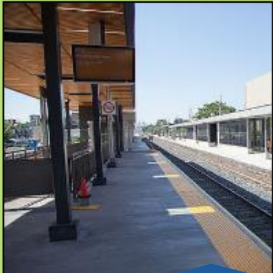
Bloor GO Tunnel (Nov 2022) Ph1 Pedestrian Diversion
