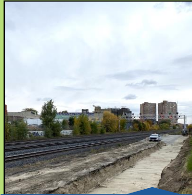
Trackbed Grading (Ongoing)
