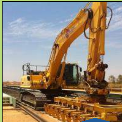
Track Work (Summer 2023)
