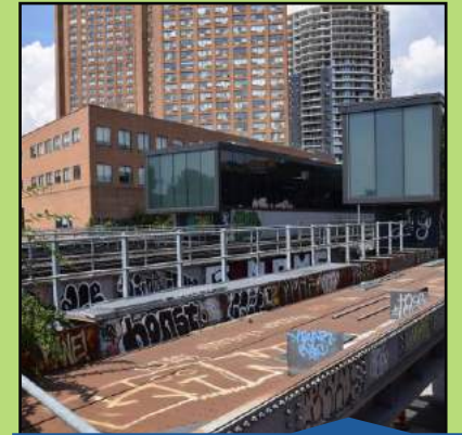
Bloor St Bridge Shift (Spring 2023)
