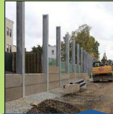
Noise/Retaining Wall Installation (Jan 2023)
