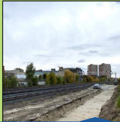
Trackbed Grading (Ongoing)
