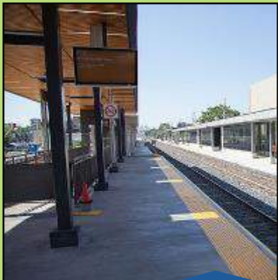
Bloor GO Tunnel (Nov 2022) Ph1 Pedestrian Diversion
