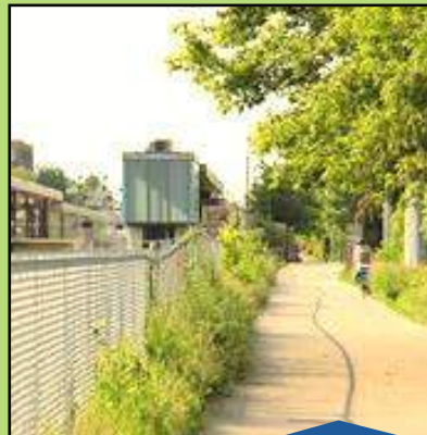
WTRP Realignment (Nov 2023) Ph2 Pedestrian Diversion
