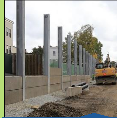
Noise/Retaining Wall Installation (Aug 2022)
