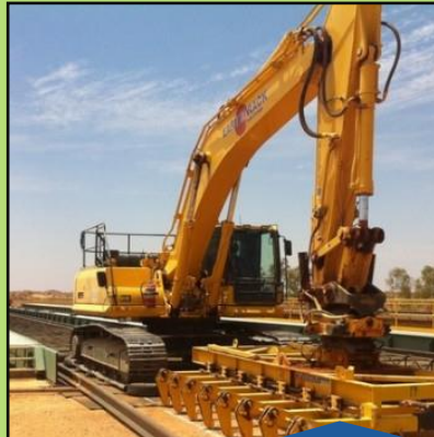
Track Work (May 2023)
