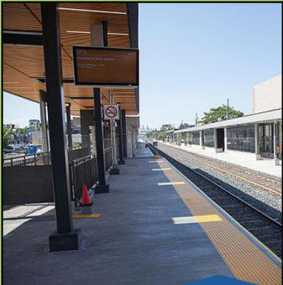
Bloor GO Tunnel (Nov 2022) Ph1 Pedestrian Diversion
