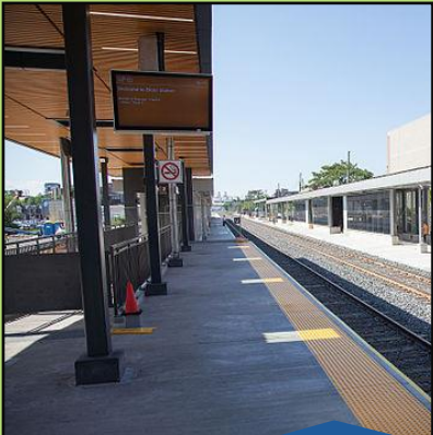
Bloor GO Tunnel (Nov 2022) Ph1 Pedestrian Diversion
