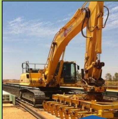
Track Work (May 2023)
