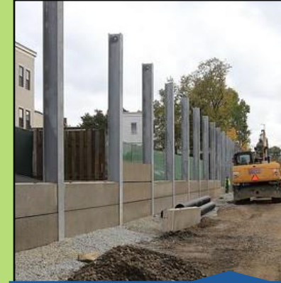
Noise/Retaining Wall Installation (Aug 2022)
