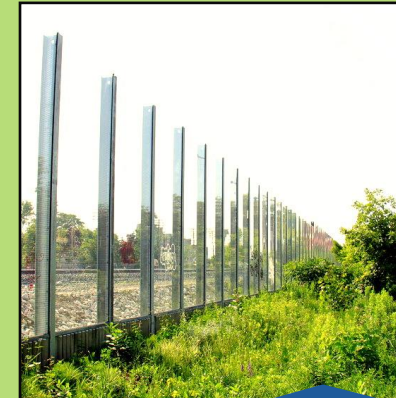
WTRP Realignment (March 2024) Ph3 Pedestrian Diversion
