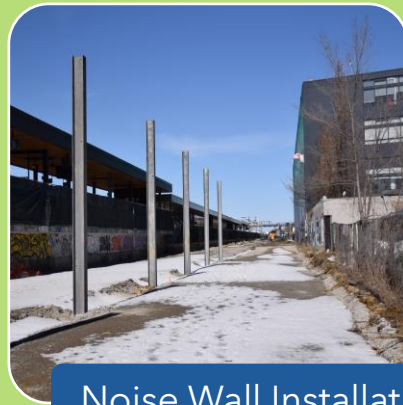
Noise Wall Installation (Ongoing)
