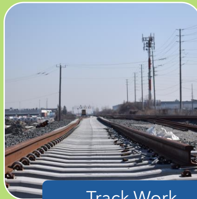
Track Work (Spring 2024)
