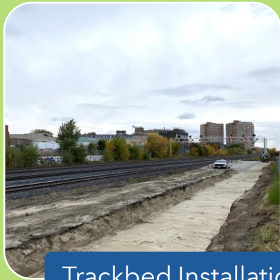
Trackbed Installation (Ongoing)
