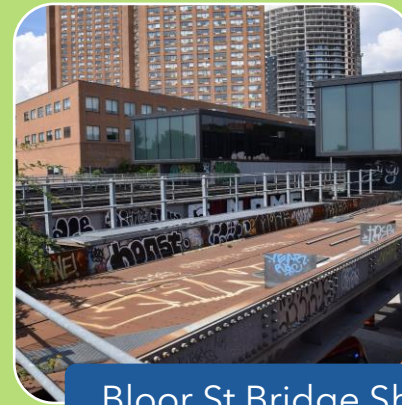
Bloor St Bridge Shift (Spring 2023)
