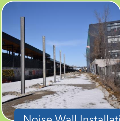
Noise Wall Installation (Ongoing)
