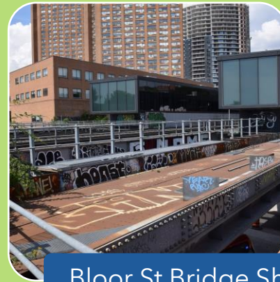
Bloor St Bridge Shift (Spring 2023)
