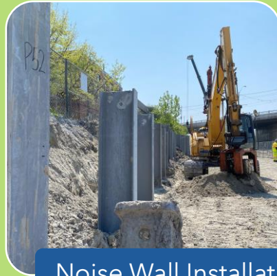
Noise Wall Installation (Ongoing)
