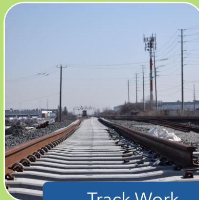
Track Work (Spring 2024)
