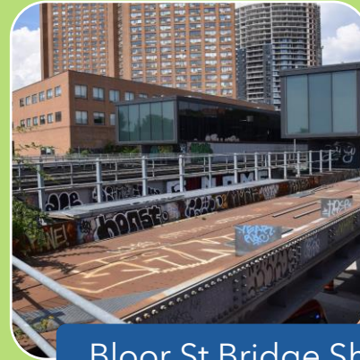
Bloor St Bridge Shift (Spring 2023)
