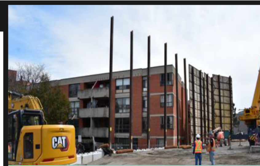
Minimizing Noise and Vibration: Scarborough Subway Extension Noise Walls
