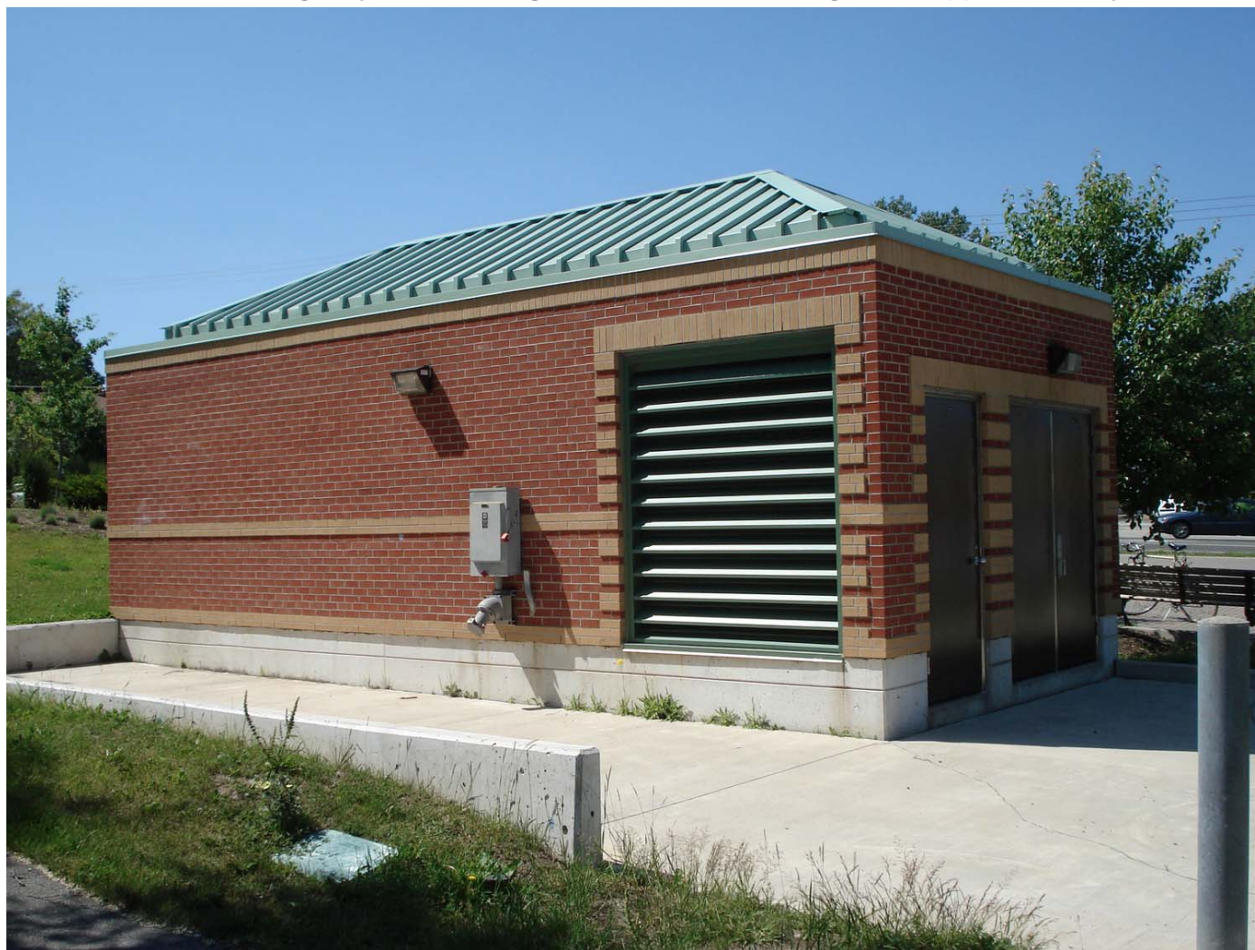
Exhibit 95: Emergency Exit Building at Bessarion Rd. Along the Sheppard subway line
