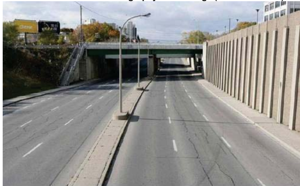
Exhibit 40: Photography Drive Bridge (Westward View)
