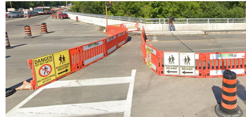
Finch/Islington (Finch W LRT) - Safe and Separated Pedestrian Detour Path
