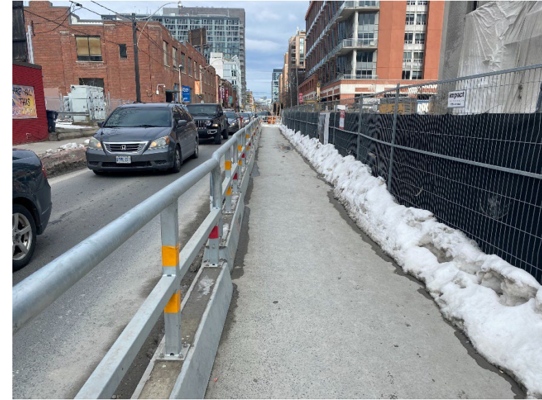
Downtown Toronto - Safe and Separated Pedestrian Detour Path
