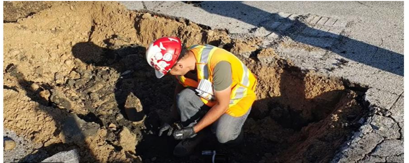
Photo: Digging test pits to test soil quality. Courtesy of Metrolinx
