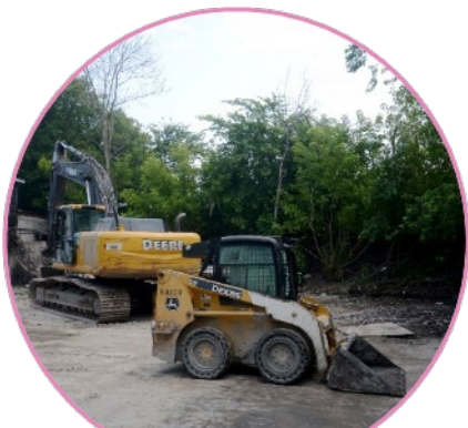
EXCAVATOR AND LOADER
