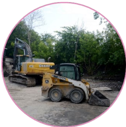
EXCAVATOR AND LOADER
