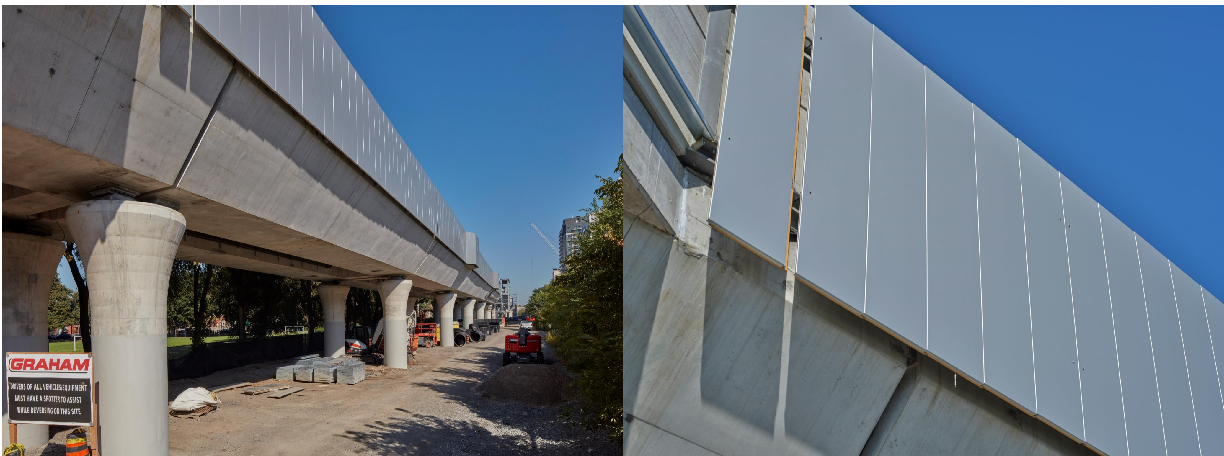
Cladding installation on the Elevated Guideway
