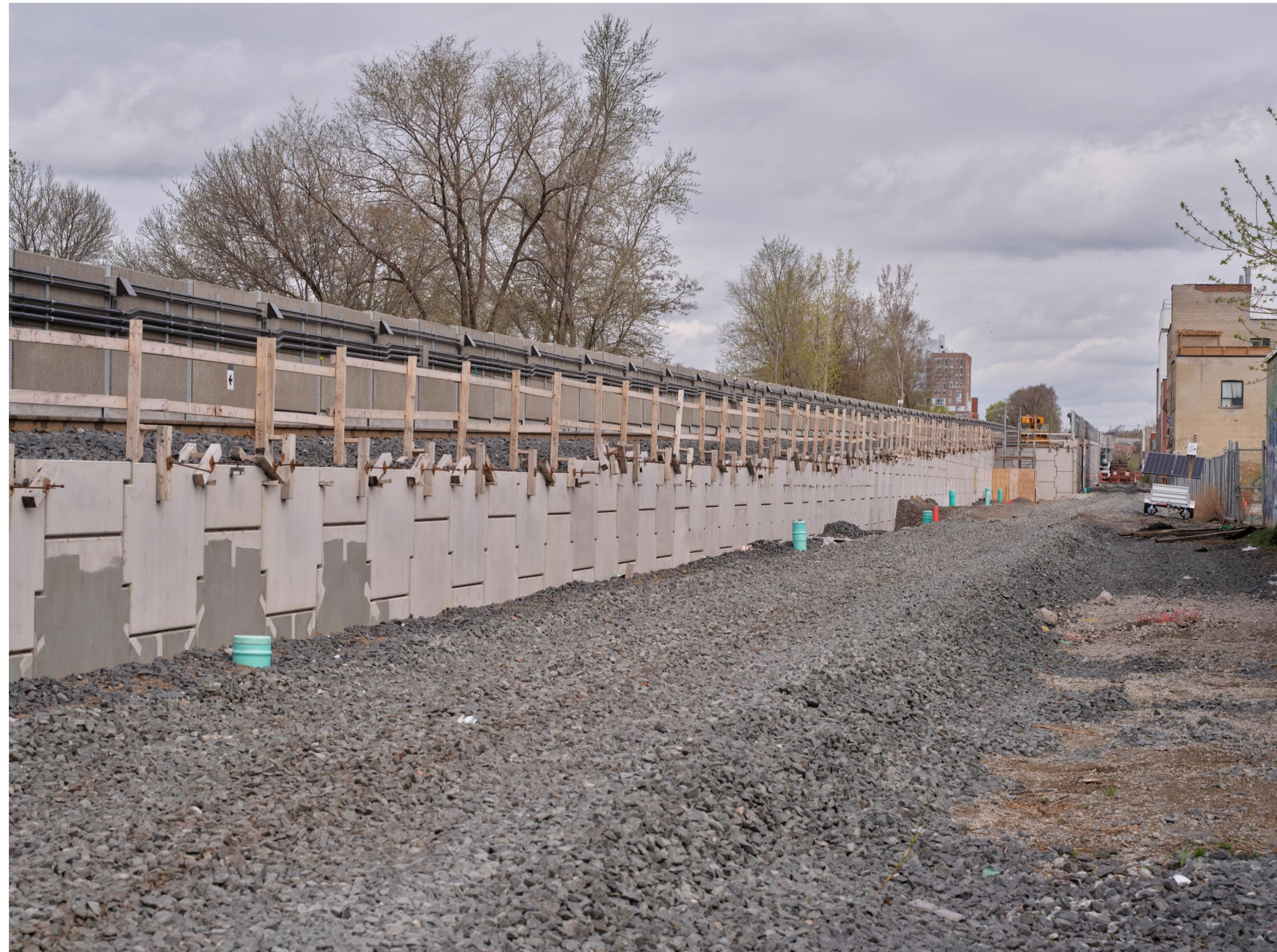
South MSE wall construction
