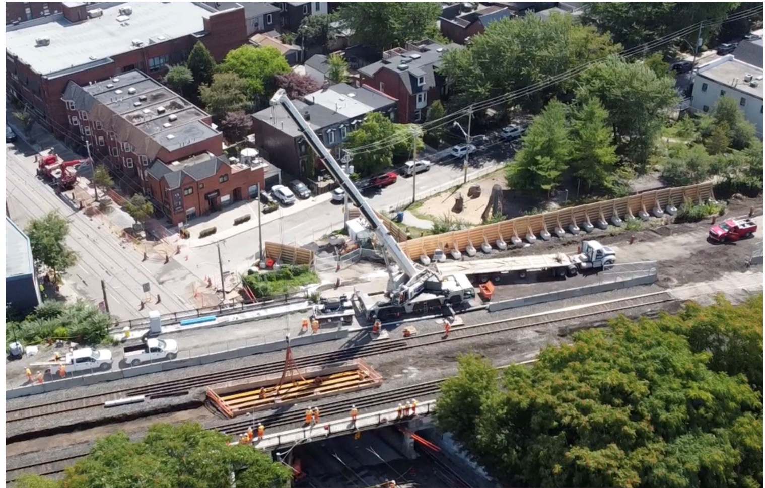
Queen St. E. Bridge Girder Installation Aug 12 - 13, 2023
