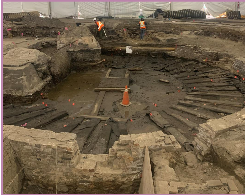
Exposed railway turntable at 271 Front Street East, facing south (above and centre bottom) - Photo courtesy of Stantec; map courtesy City of Toronto
