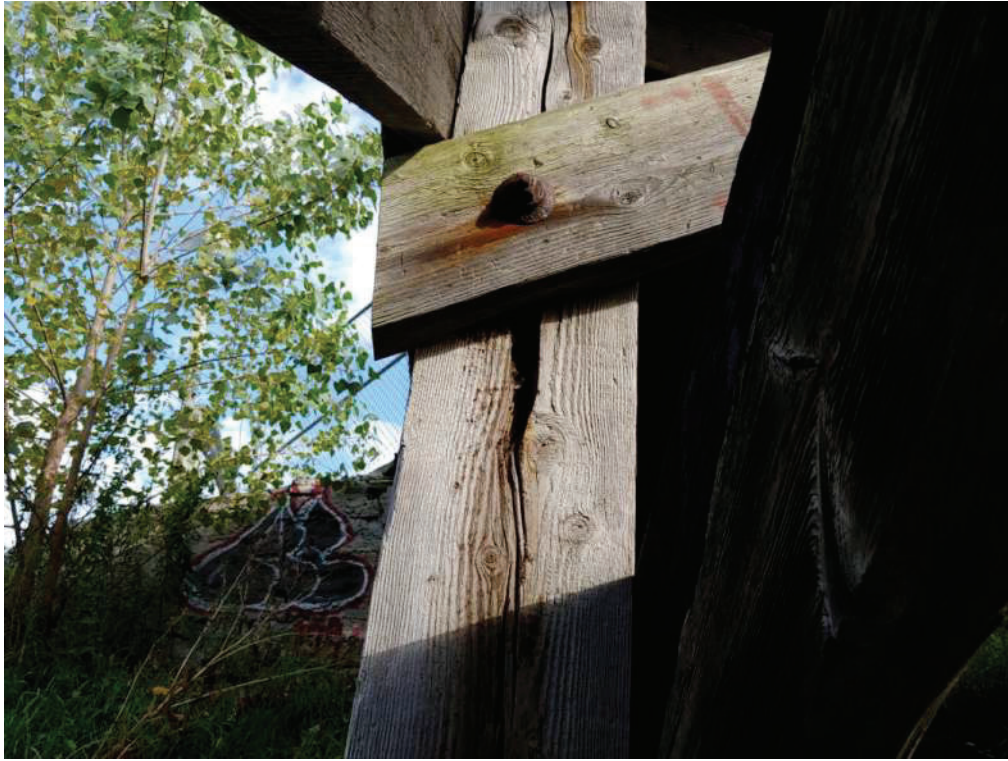
Image 13 – Split timber beam at north pier (looking north)
