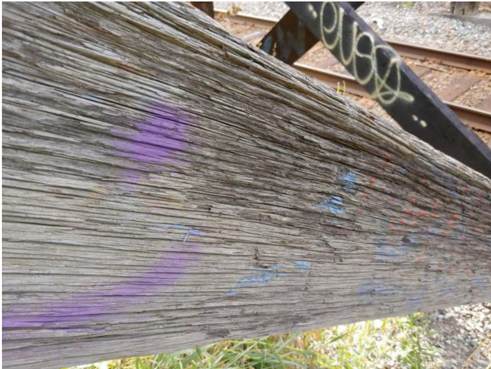
Image 14 – Heavy weathering on timber beam (typical)
