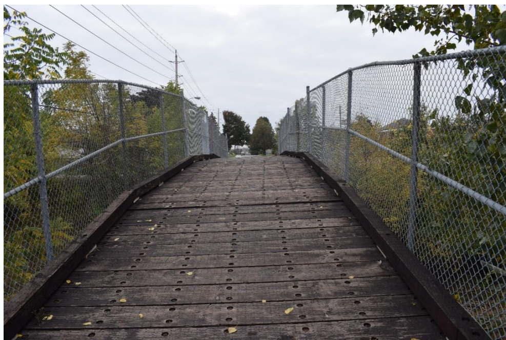
Plate 20: Laminated bridge deck, curb, and fence, looking south
