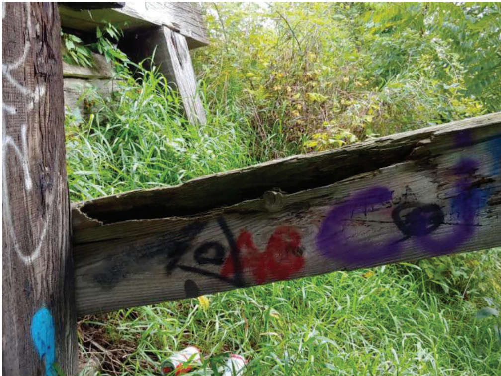
Image 12 – Timber rot at north abutment (looking east)
