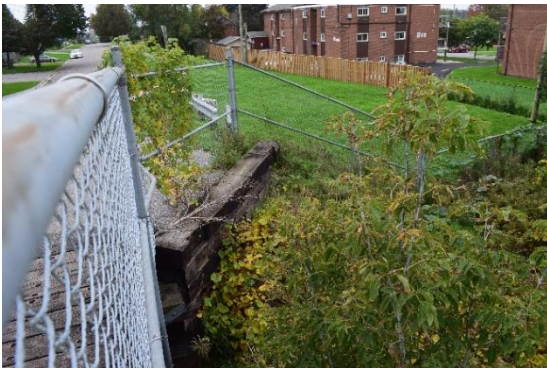
Plate 9: Timber wingwall, looking southwest
