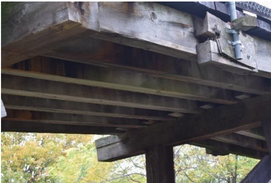
Plate 7: Longitudinal timber floor beams, looking east
