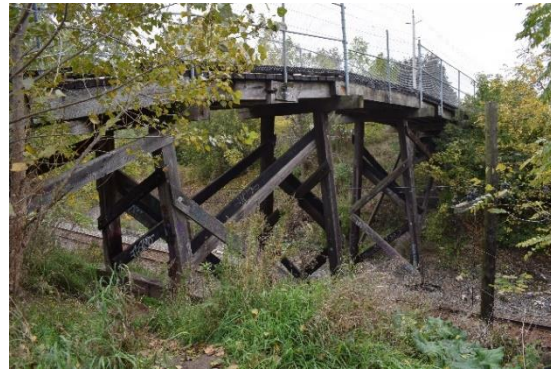
Plate 8: Transverse beams and piers, looking southeast
