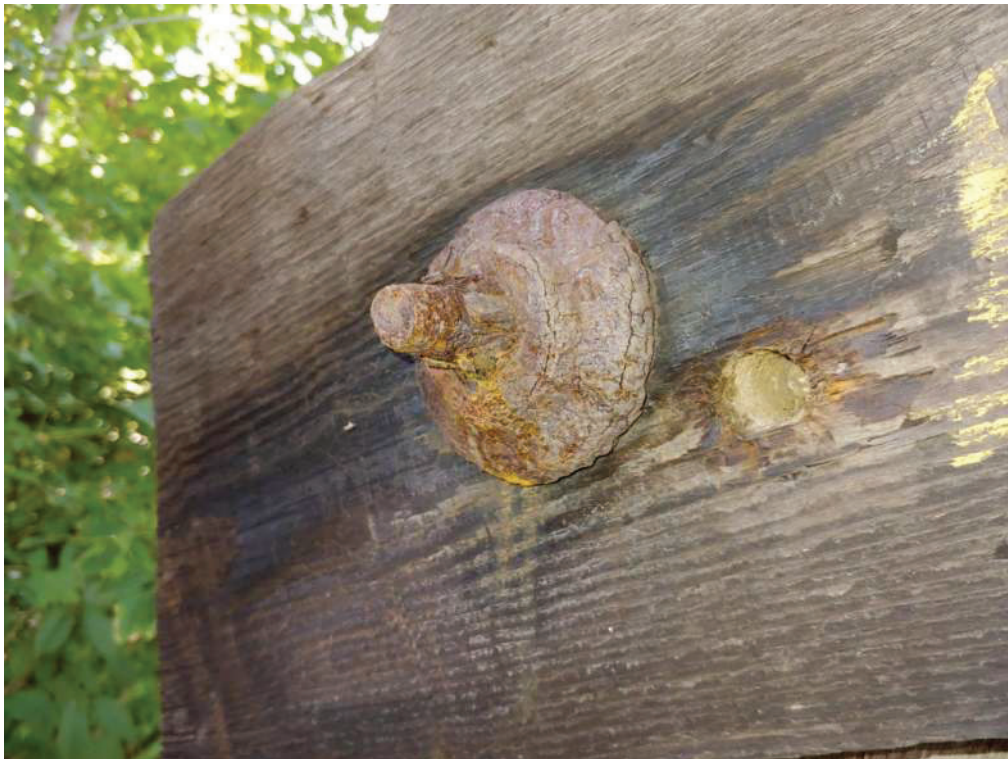
Image 16 – Severely corroded bolt (typical)
