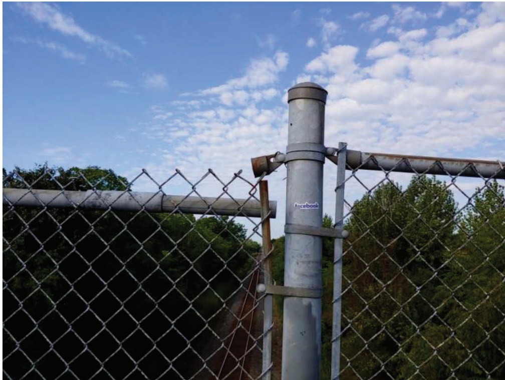
Image 10 – Disconnected fence section
