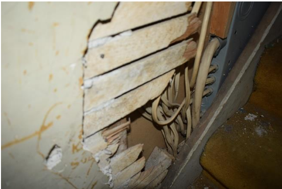
Photo 36: Lath and plaster, looking north
