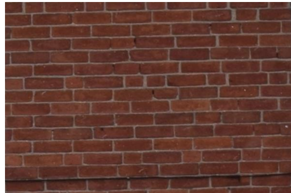
Photo 3: Common bond brick with Flemish header details, looking west
